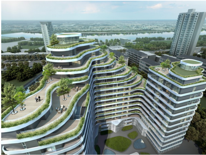
Shanghai Weifang Village Street project, Pudong District
