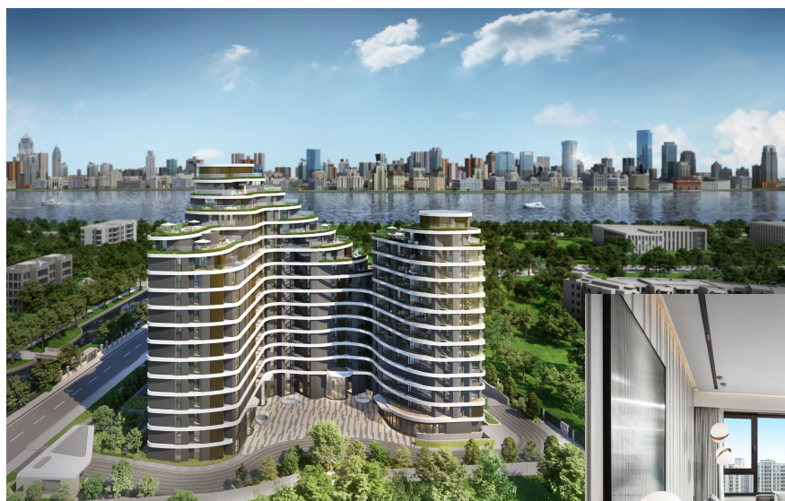
Shanghai Navale, Pudong New District
