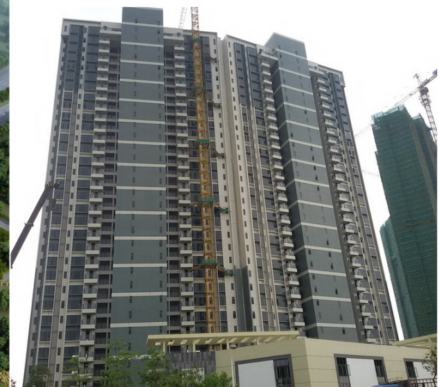
Phase 2 progress as of Jul 2015
