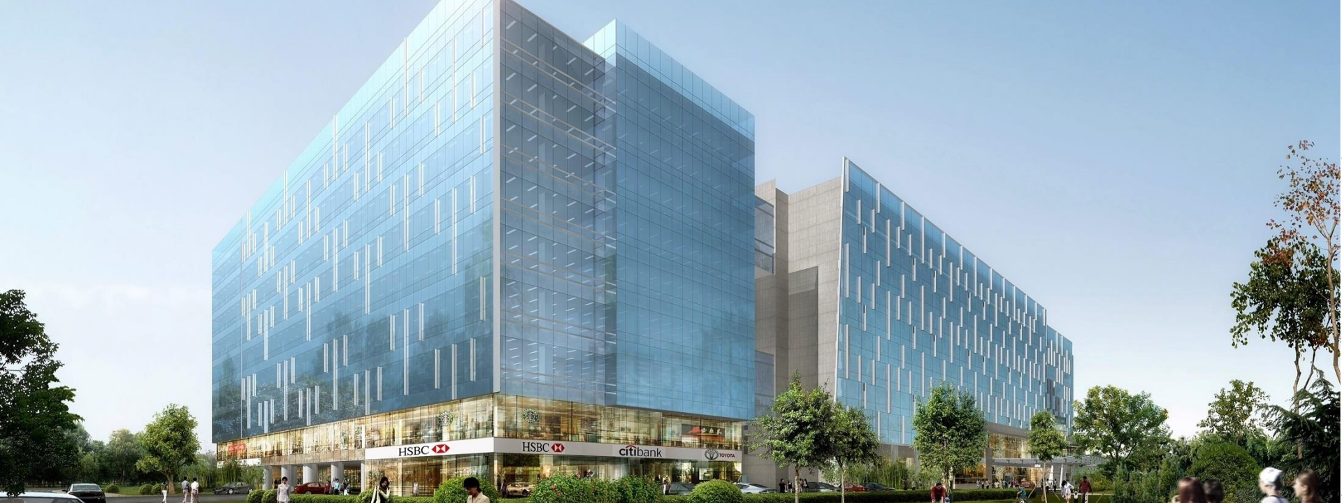
Huadu Jiahua Plaza Phase 3 , Guangzhou
